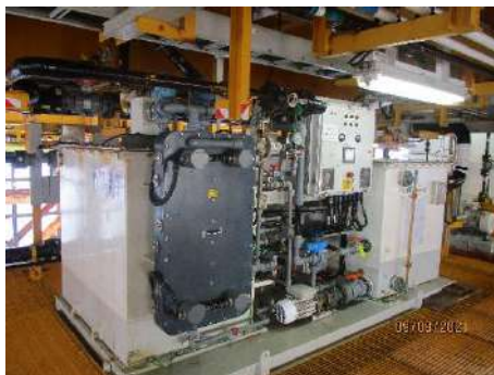
Figure 2-8 Sewage treatment system
