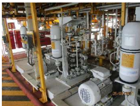
Figure 2-6 Wastewater treatment system
