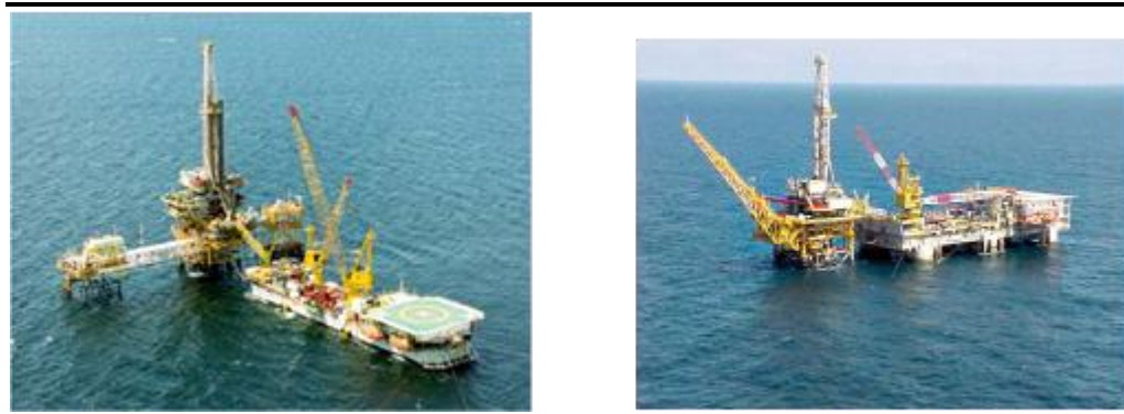
Figure 1.4 Example of Tender Assisted Rigs
