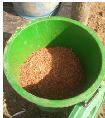
Figure 2-6 Drip pan and absorbent material.
