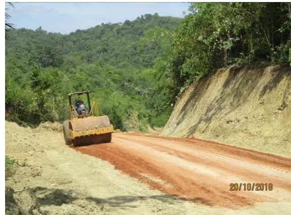
Figure 1-2 Moenatkone (MNK) Wellsite in Site Preparation and access road construction
