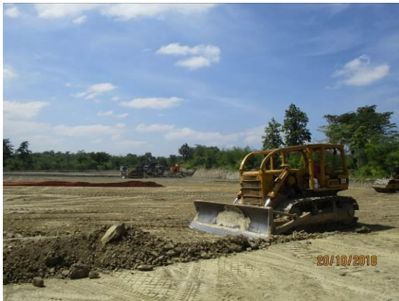
Figure 1-2 Moenatkone (MNK) Wellsite in Site Preparation and access road construction
