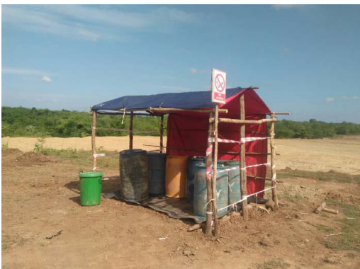
Figure 2-6 Drip pan and absorbent material.
