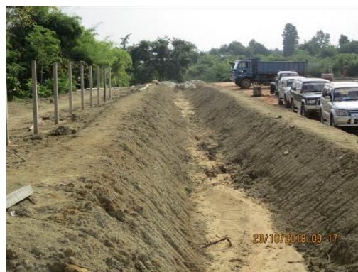
Figure 2-7 Water drainage around the well site.
