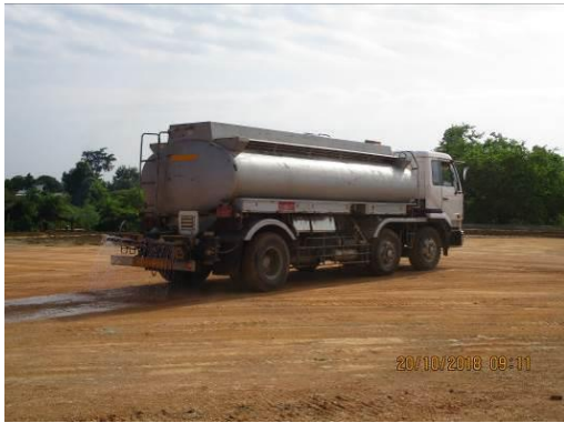
Figure 2-2 Water Spray within construction area and the access road.
