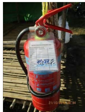
Figure 2-19 Inspection of fire extinguishers
